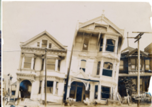
Evidence of earthquake
